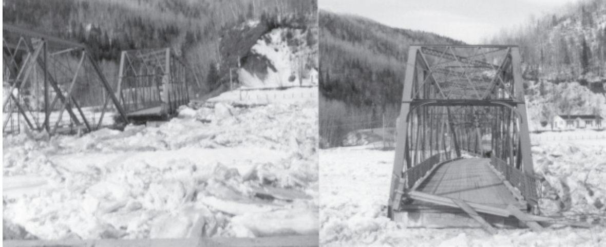
St-Alexis Bridge (standing at 24 feet above normal water level) engulfed in ice during the 1994 flood, to be later totally destroyed. (Notice in picture on the right how bridge is bent)
